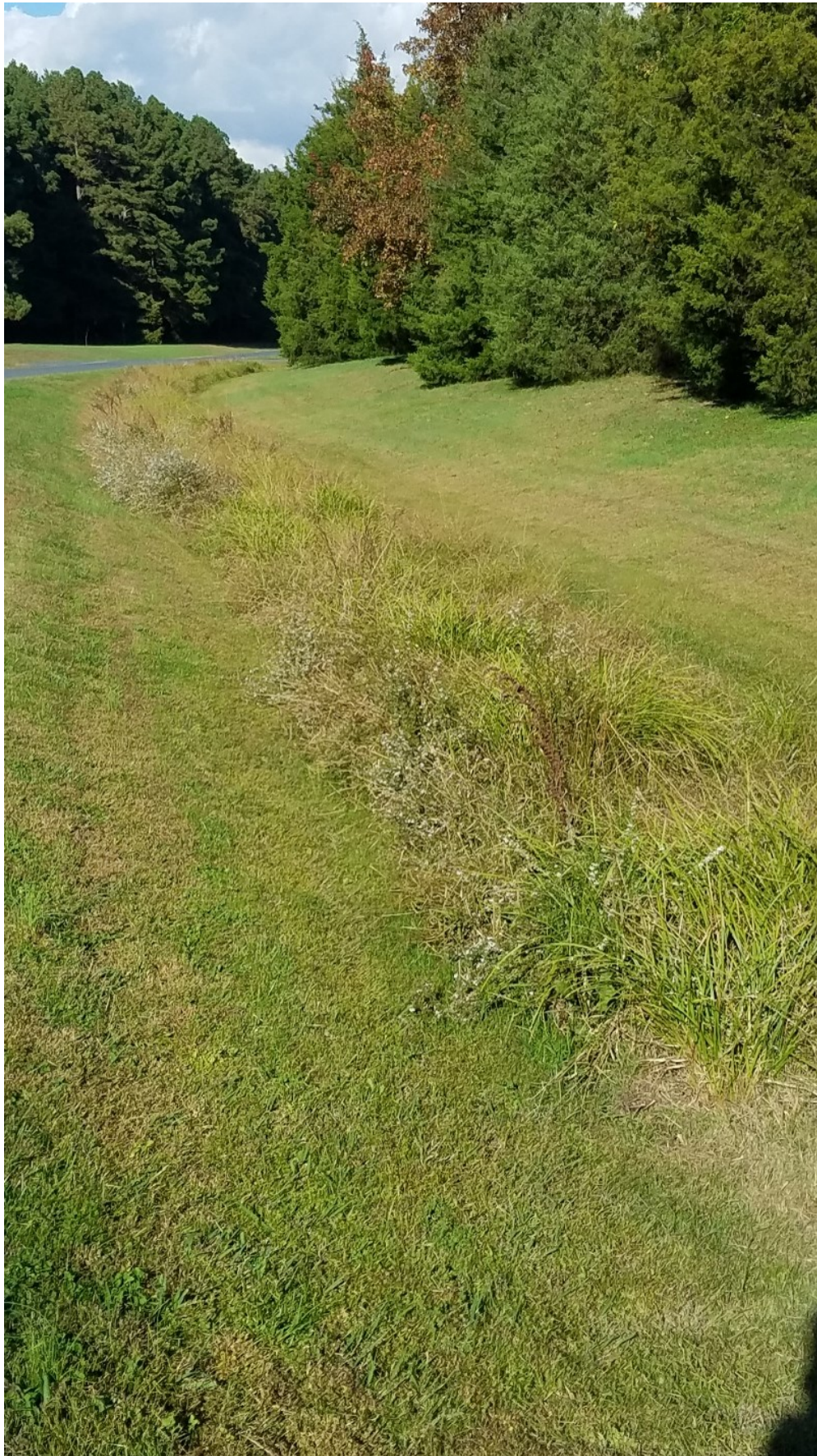
Overgrown Drainage Ditch
